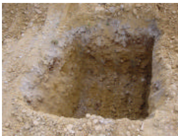
Solera a compactar
