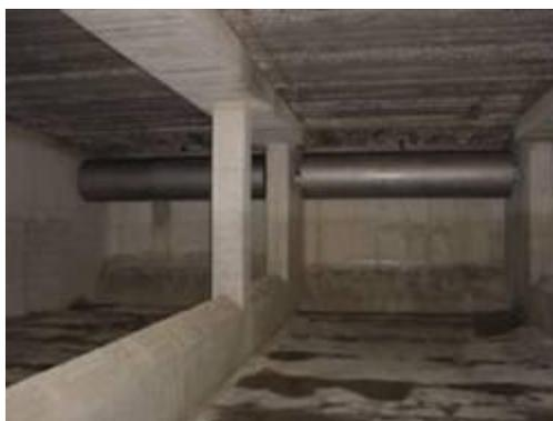
Figure 3: Low-wall lane separation.
