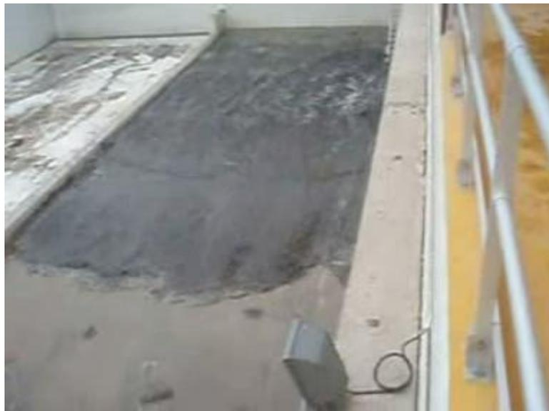
Figure 1: Cleaning wave generated by the vacuum system discharge.
