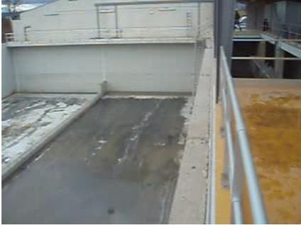
One of the problems presented by storm tanks is that, after a rainy event in which the wastewater is retained inside, sedimentation occurs from part of the solids that accompany it on the surface of the retention chamber. This sedimentation can cause problems of odors and loss of healthiness in the facilities, so it is imperative to eliminate it.
