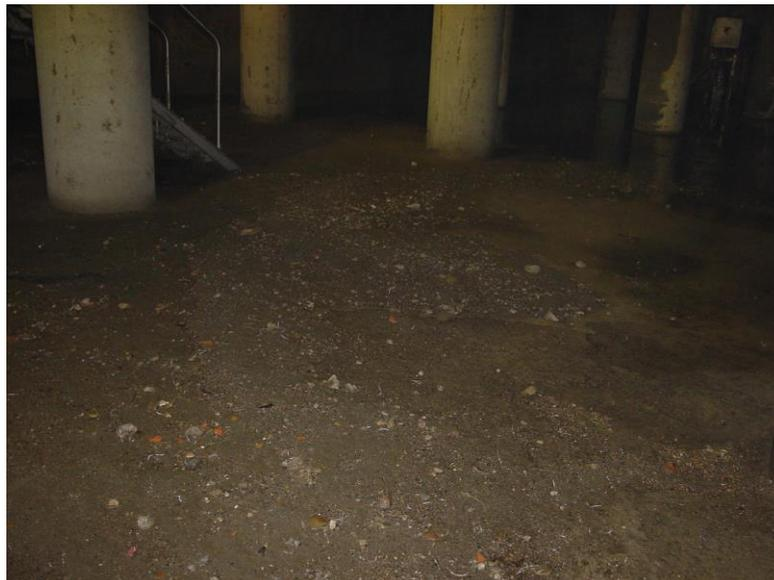
**Fig. 1. Sedimentation in storm tank.**
