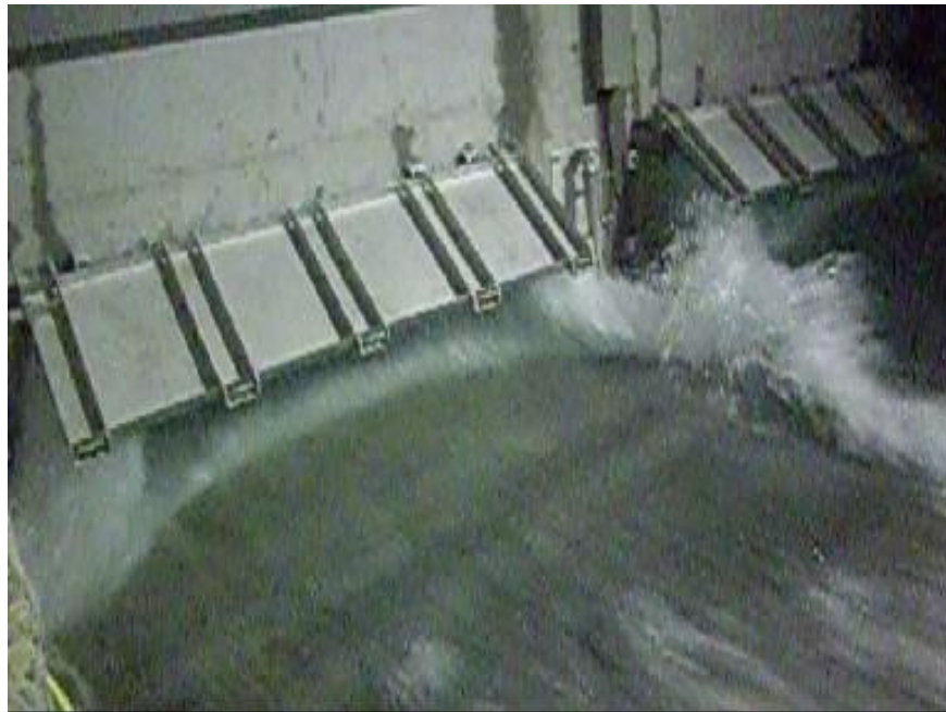
Image: Discharging the flushing chamber
